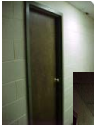
Above: New solid core doors were stained and hung throughout the house.
